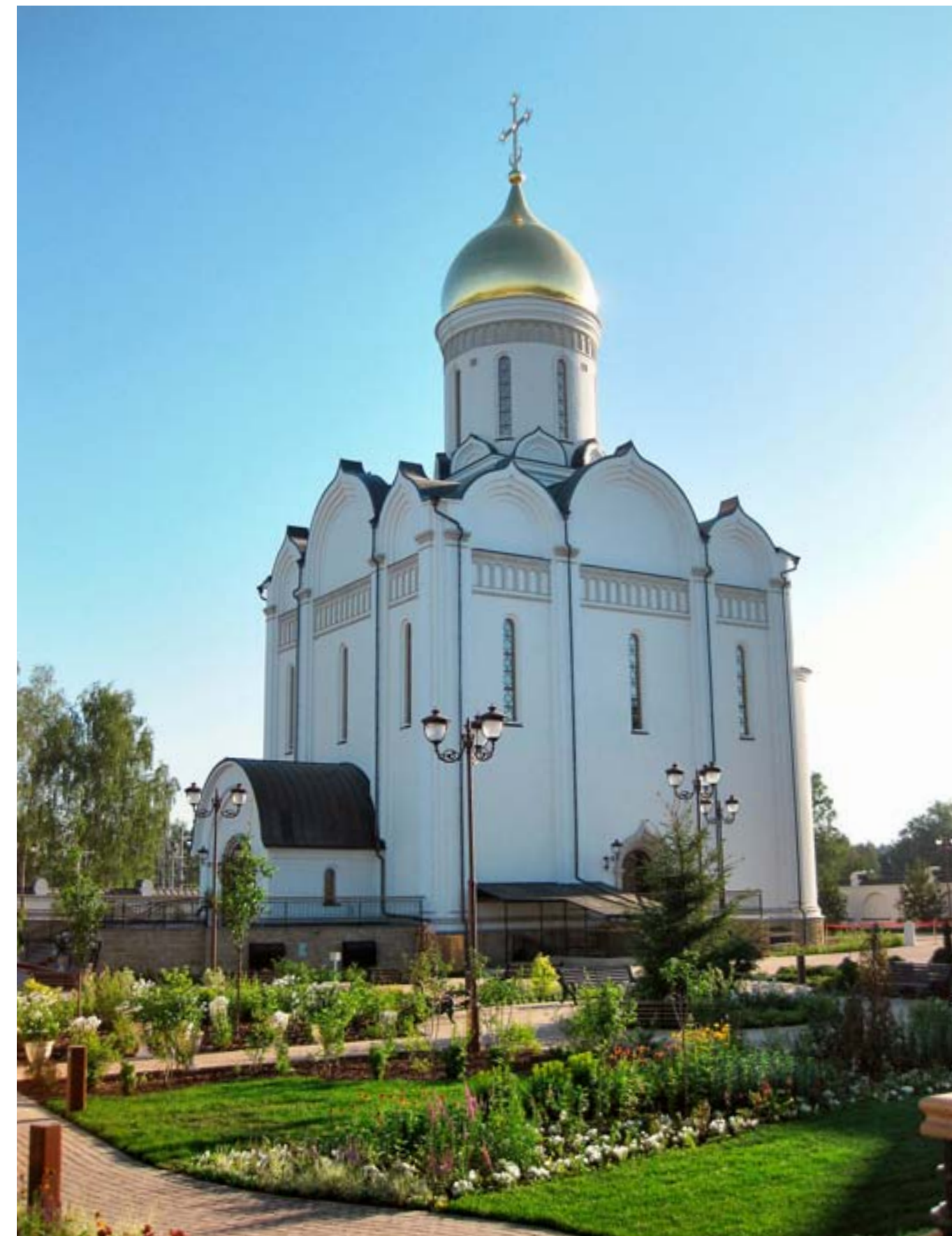
The construction of the Orthodox temple in Usovo village (Moscow region) was financed by Rosneft.
